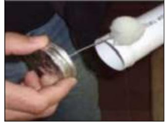
*Always glue the pipe, not the fittings, to prevent excess glue residue.*
