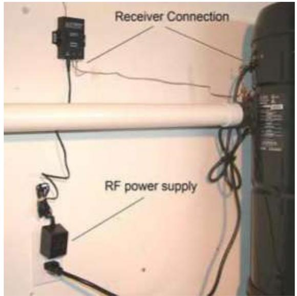
**NOTE:** When locating a radio-frequency (RF) receiver by a central vac power unit that operates on 240V, please request an additional 120V receptacle for the RF receiver – it does not need to be a dedicated circuit.
