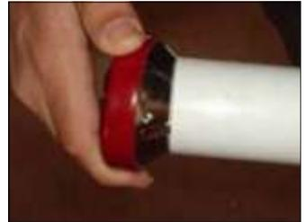
*Use a deburring tool (or other tool) to remove all burrs from pipes.*
